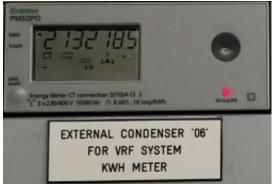
The Optergy Proton controller can use the existing pulse meters by installing counter modules. This would considerably reduce the initial costs and still offer all the benefits of the Optergy Proton system. However as mentioned above pulse meters can easily become out of sync from the actual readings and should therefore be regularly checked and calibrated.
